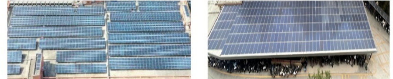
Distributed Power Stations
